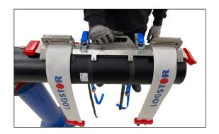
Install the pressure tool straps loosely around the joint.
