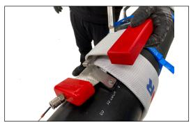
Wrap the pressure band around the sleeve and pull, so that the pressure band is in contact with the sleeve.
