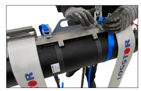
Push the pressure tool upwards from the bottom until stop against the rubber rail on the steel rail, so it is aligned with the edge of the overlap.
