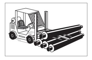
Carefully lift the pipes off the lorry trailer with the forklift.
