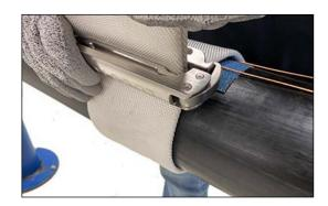
Push the wedge between the pressure band and the AirLock. Make sure the wedge is installed in the middle of the pressure band.
