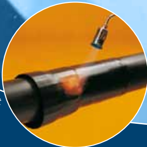
Heating the BXSJoint Second seal
