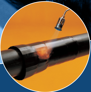
Shrinking the BXJoint sleeve. Second seal
