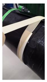
As an alternative to masking tape, teflon band can be used. Teflon band is reusable. It can be ordered from LOGSTOR, product number 9000000041000.
