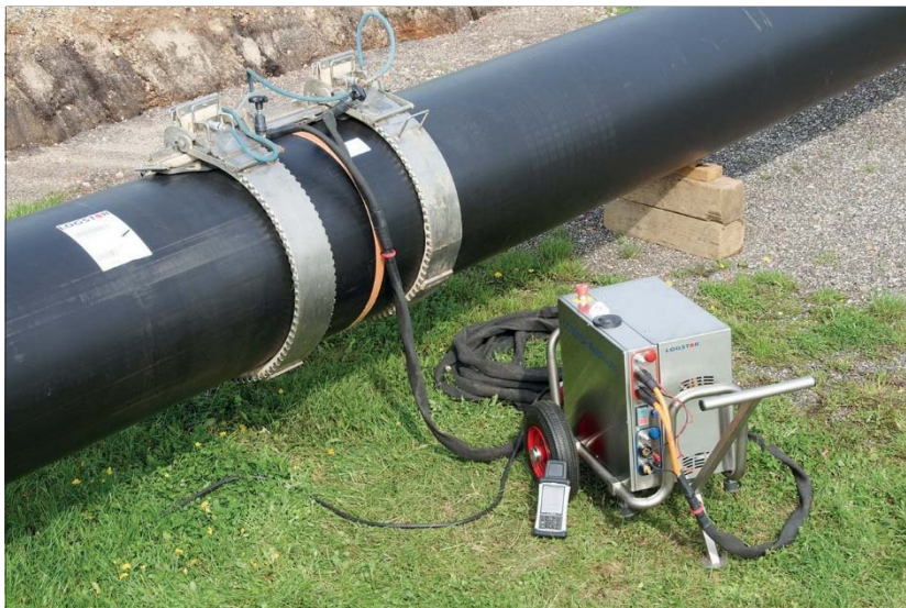
Figure 5. The LOGSTOR Weldmaster is a multifunctional PE welding device which allows for quick and secure installation of the casing joint
