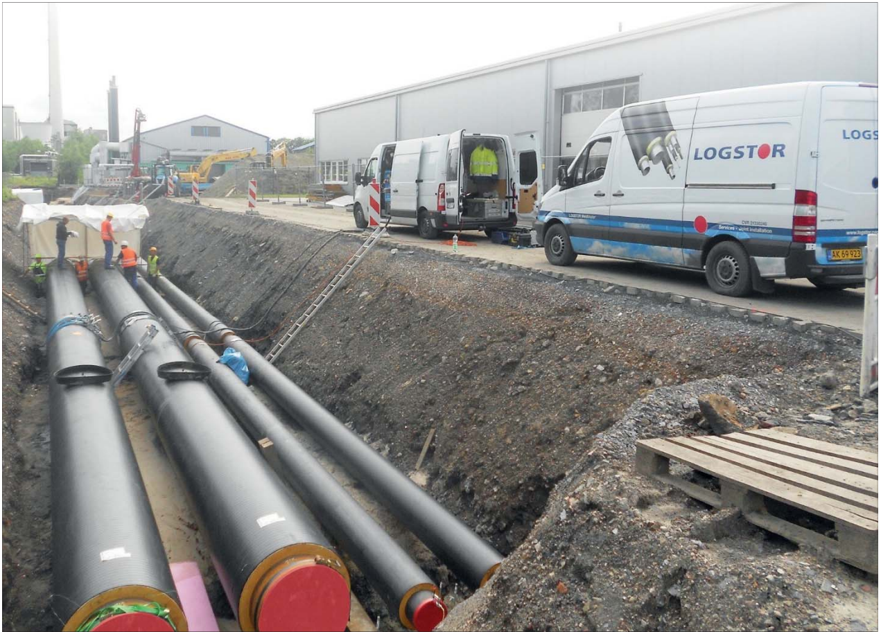
Figure 4. Installation of the LOGSTOR PlateJoints on the pipelines
