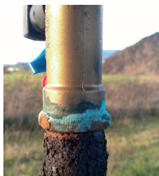
Fig. 3 - Released copper ions from brass valve, causing corrosion of the steel pipe. The damage is on the return pipe. No damage on the flow pipe.
