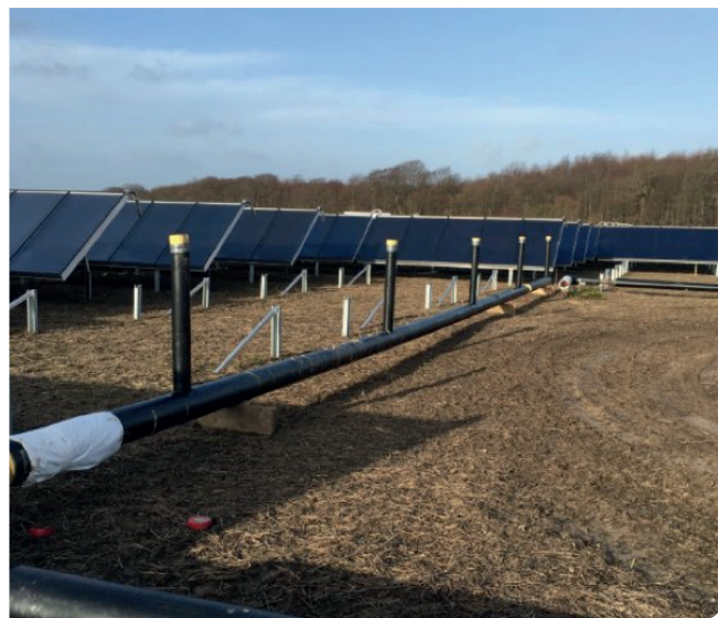
Fig. 8 and 9 - Standpipes made indoor. In the indoor factory, straight pipelines are manufactured with standpipes, designed so they match the exact position of the solar panels.
