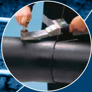
Welding plugs are fitted and welded
