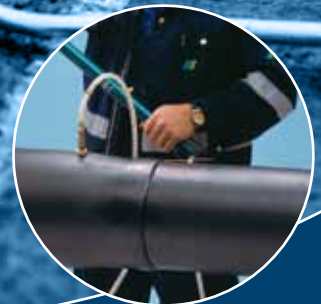
Testing the seal prior to foaming
