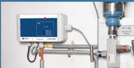
*The surveillance unit X4 is used for resistance and impedance measurements.*
