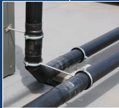
The pipes are jointed with press couplings, encased in PUR insulating shells and 100% sealed with shrinkable joints.
