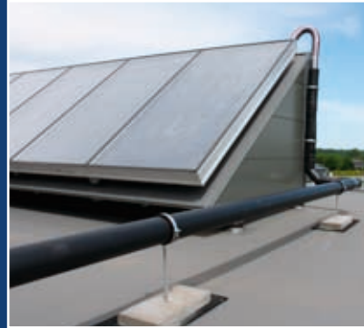
The straight pipes are available in 5 meters for copper pipes and 6 meters for electroplated steel pipes.
