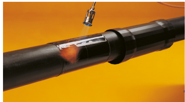
Shrinking the shrink film. First seal
