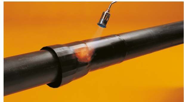
Shrinking the BXJoint sleeve. Second seal
